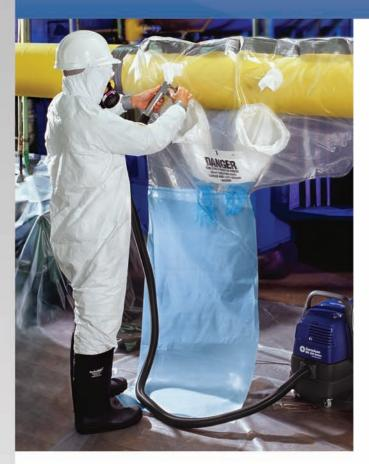
The QuickTwist glovebag design will allow removal of up to 50% more linear footage of asbestos per bag than the old standard glovebag.
